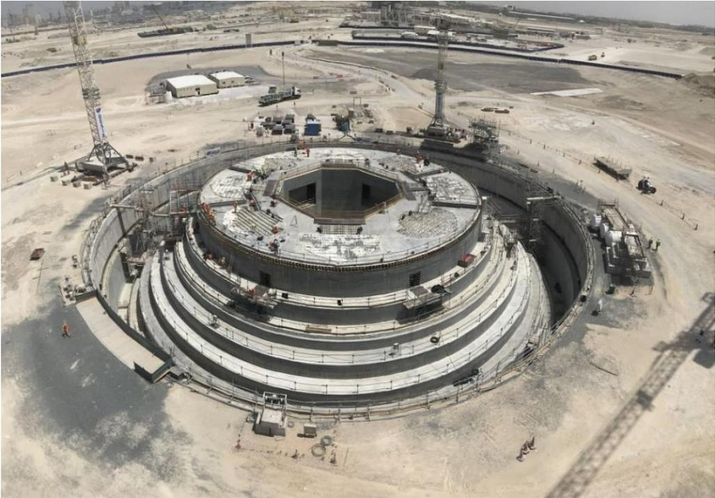
Figure 2.2 Dubai Creek Tower's pile cap, [66].
